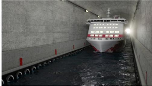
Norwegian officials have given the green light to fully finance what is set to become the world's first full-scale ship tunnel, bypassing one of the most dangerous areas for vessels along the Norwegian coast. The Stad Ship Tunnel will be blasted through 1.7 kilometers of rock at the narrowest point of the Stad Peninsula, allowing ships the size of Hurtigruten's coastal steamers to navigate it.
